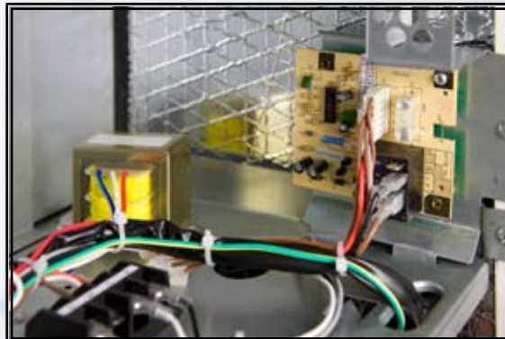
24V Transformer, Time-Delay Relay & Smart Diagnostics PC Board
